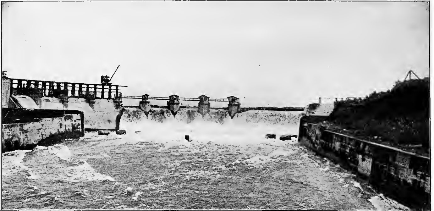
THE SPILLWAY AT HIGH WATER
